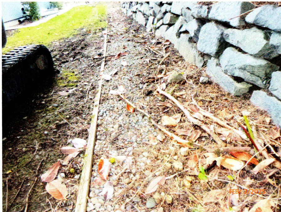
REAR YARD DOUBLE ROCKERY AND BASE "FRENCH DRAIN"
