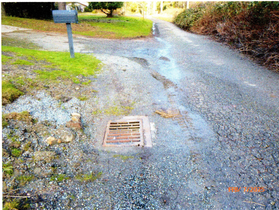
EXISTING CATCH BASIN ON 97TH AVENUE S.E.
