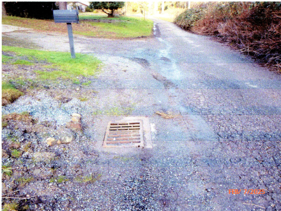
EXISTING CATCH BASIN ON 97TH AVENUE S.E.
